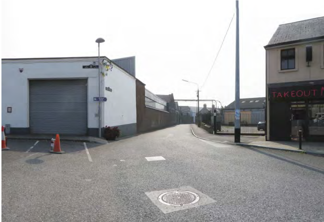
Fig 23: View of New Road showing a lack of active frontages and visual clutter providing a poor public realm.
